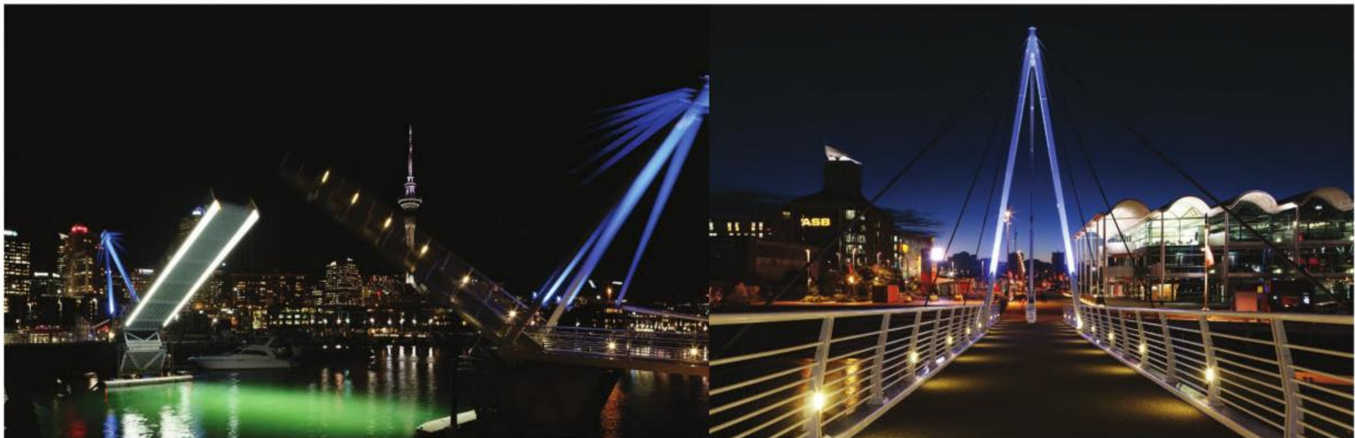
Safety and aesthetics go hand in hand on the Wynyard Crossing Bridge in Auckland.
